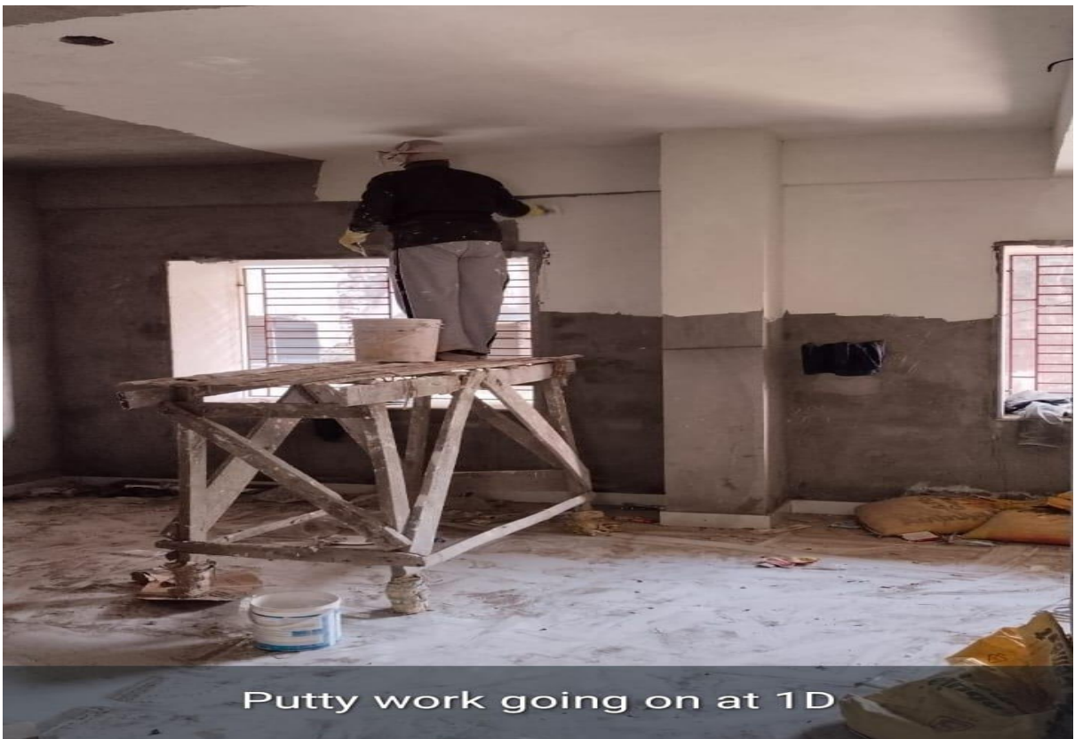
Putty work going on at 1C
